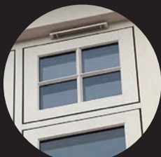
Trickle vent through the Flush Sash outer frame
